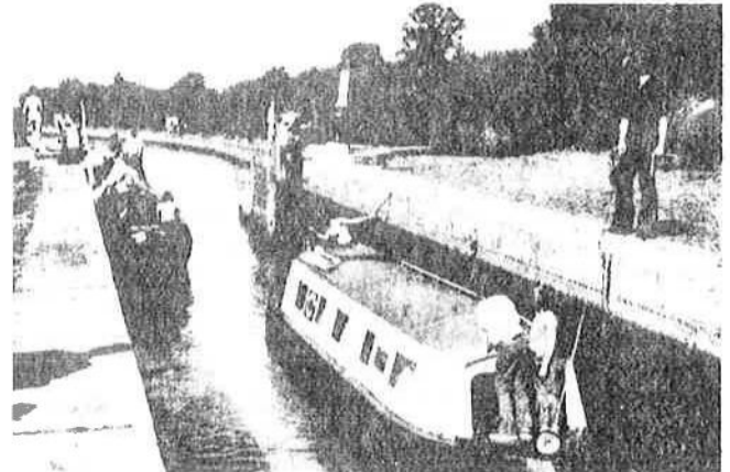
Plate 10.15 Calcutt lock (Grand Union Canal) showing safety chains. (PFP)
